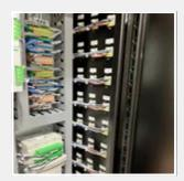
Industrial processes and infrastructures are controlled and secured via control cabinets. With the Han® Protect, HARTING has developed a new connector that simplifies protection and reduces the required installation space in the control cabinet. Blown fuses can be detected by LED without opening the cabinet and replaced without tools.
